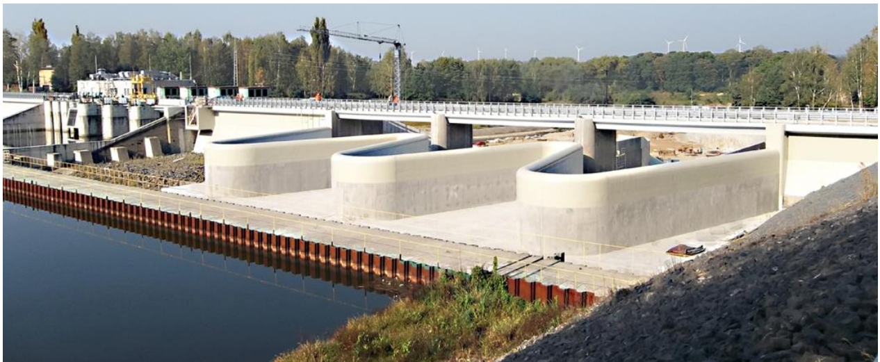
Figure 1: The Niedów dam after reconstruction (fot. Wojciech Rędownicz)
