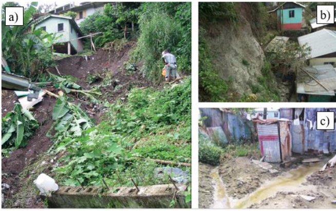
720 Figure 1: Examples of informal housing affecting land stability. The image (a) and (b) show examples of unsupported cut slopes, respectively in Saint Lucia (Caribbean) and Dumsi Pakha (K Kalimpong, India). The image (c) shows the effect of lack of water management in an informal community of Saint Lucia (Caribbean). From the blog AGU landslides: https://blogs.agu.org/landslideblog/2016/03/14/managing-urban-landslides-1/ and the community based project Mosaic (Anderson and Holcombe, 2013)
