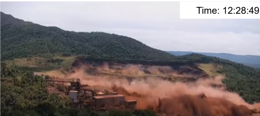
Figure 3: Stills from the YouTube video of the Brumadinho dam failure
