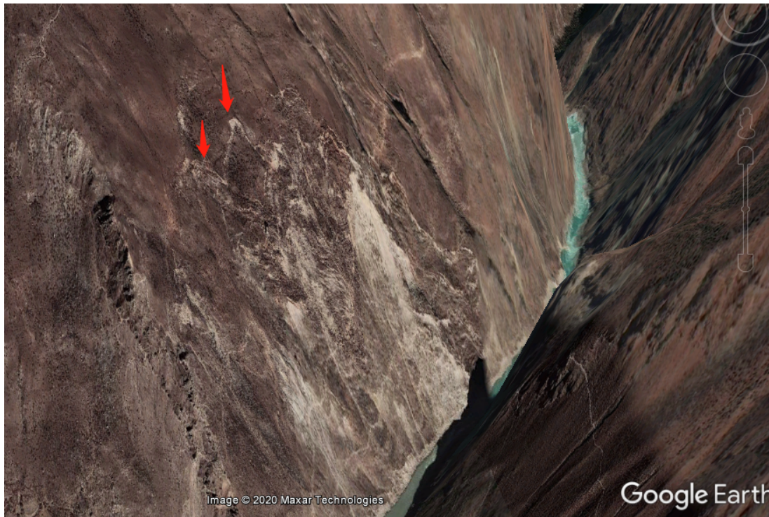
Fig. 1. 3-D view of the Mindu slope in Google Earth. Red arrows indicate tension cracks as the slope moved down. Light colour on the slope indicate fresh exposed substrate.
