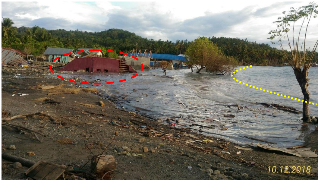
10 Figure 12: Quick landsubsidence in Lero Village. Photograph taken two weeks after the event. Some houses dropped suddenly, around 3-4 m, when the earthquake occurred. Residents of these houses, especially that indicated by the oval, could not save themselves. The yellow dotted line is the former coastline.
