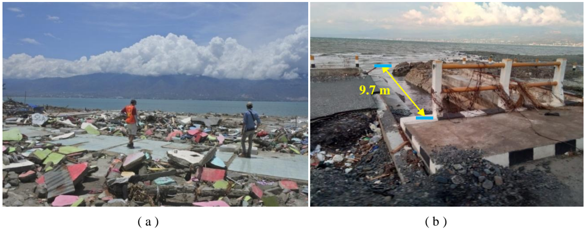
Figure 6: (a) Damage caused by the tsunami in Tondo, a residential complex where a lot of private boarding houses were inhabited by students at the University of Tadulako, and (b) a reinforced concrete bridge on Cumi-cumi Road Palu City shifted by 9.7 m by the tsunami.
