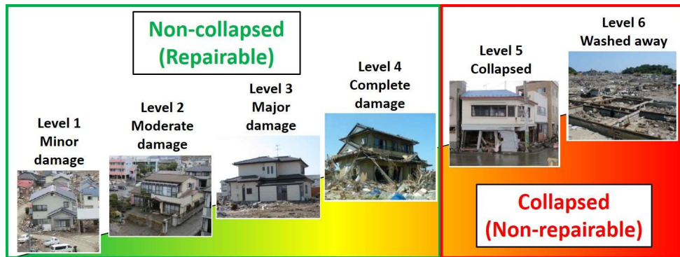
182 183 Fig. 3 Building damage levels and collapsed condition considered in this study. 184
