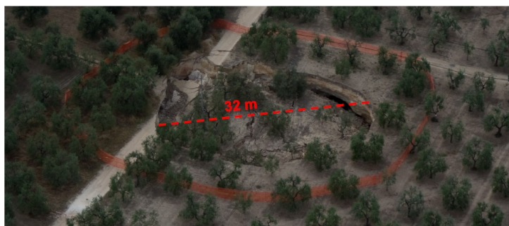
165 166 Figure 5. Aerial view of the sinkhole occurred in the Barletta area.
