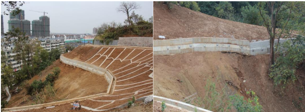
(a) Original supporting structure (b) Cracks in antislide piles
