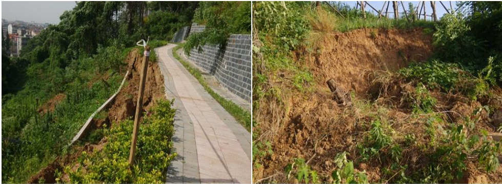
(c) Downhill scarps and tension cracks at the rear edge of the slope
