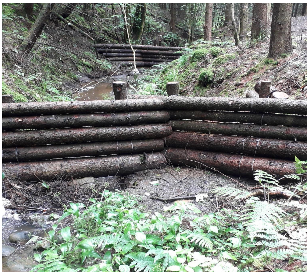
Figure 1: Leaky barriers in sequence in Penny Gill, Cumbria (B. Hankin)
