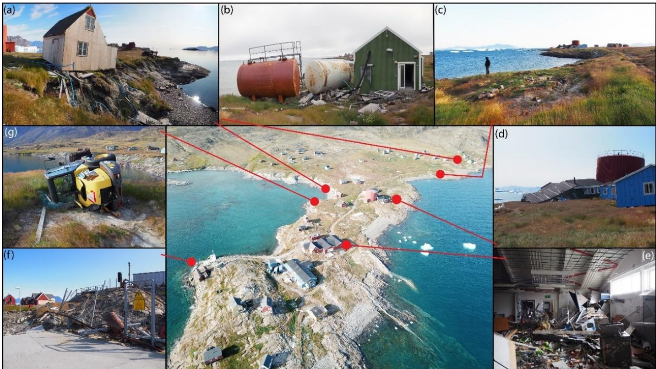
605 Figure 8. Examples of infrastructure damages caused by 2017 tsunami in Nuugaatsiaq. (a) Wooden house removed by wave from point foundation transported several dozen of meters; (b) Fuel tanks washed away from concrete frames and pushed towards power plant. Note large accumulation of litter and tsunami deposits around and inside the buildings; (c) site of former building position, which was destroyed and swept away by tsunami. Note broken wooden point foundations, media connections and erosional gullies; (d) Smashed and collapsed wooden school building moved towards major water tank; (e) Interior of local shopping centre passed by tsunami. Note large amounts of litter and rotting food supplies and twisted and bowed metal frame construction; (f) Partly-torn metal fence around fuel storage site which acted as a trap for litter transported by tsunami; (g) example of heavy machine knocked over by waves. 610
