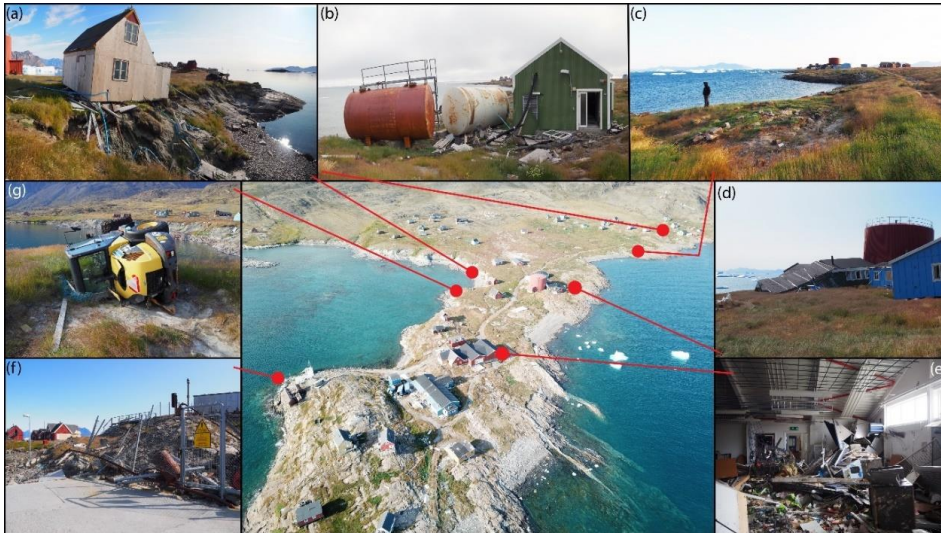
Figure 7. Examples of infrastructure damages caused by 2017 tsunami in Nuugaatsiaq. (a) Wooden house removed by wave from point foundation transported several dozen of meters; (b) Fuel tanks washed away from concrete frames and pushed towards power plant. Note large accumulation of litter and tsunami deposits around and inside the buildings; (c) site of former building position, which was destroyed and swept away by tsunami. Note broken wooden point foundations, media connections and erosional gullies; (d) Smashed and collapsed wooden school building moved towards major water tank; (e) Interior of local shopping centre passed by tsunami. Note large amounts of litter and rotting food supplies and twisted and bowed metal frame construction; (f) Partly-torn metal fence around fuel storage site which acted as a trap for litter transported by tsunami; (g) example of heavy machine knocked over by waves.
