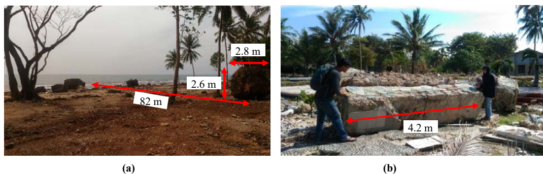
Figure 8: (a) Boulder that moved around 82 m inland and (b) an element of seawall that moved around 30 m inland.
