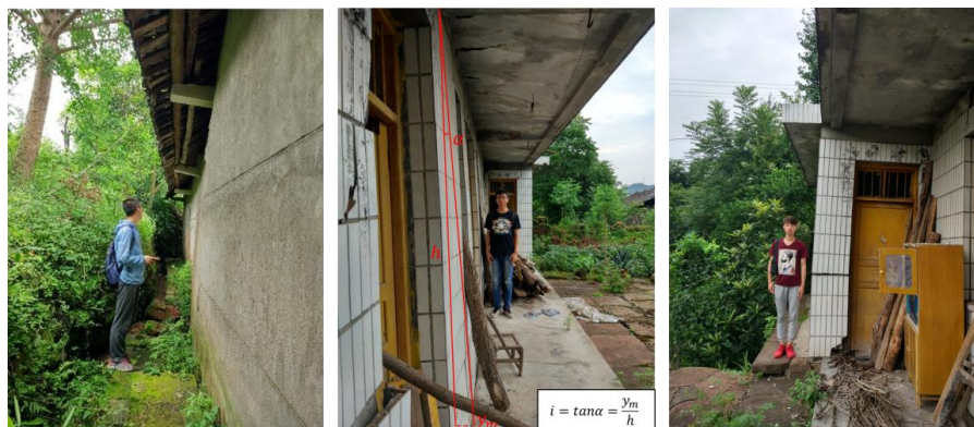
Fig. 9. The integral decline state of the object building.
