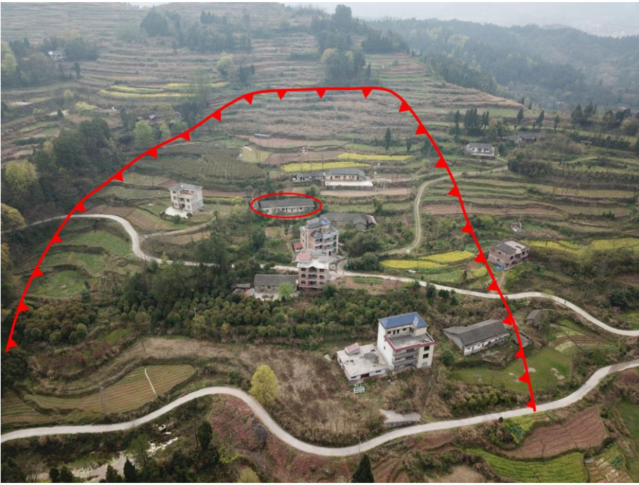
Fig. 8. A typical example of a damaged building in the landslide area (Unmanned Air Vehicle image obtained during field investigation ).
