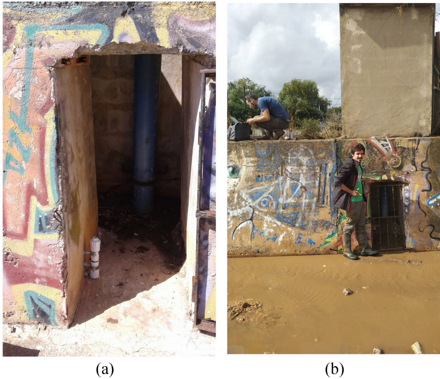
Fig. 2. Hydrometric station of the Begura de Saumà River. (a) Installation of the digital equipment, 10th June 2015. (b) Data downloading the day after the flash-flood -10th October 2018-.
