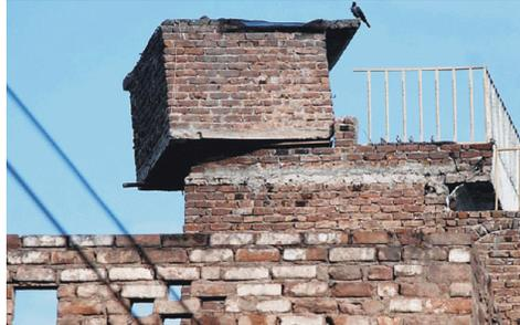
(b) Peshawar City, Ganj: Sliding of overhead tank on the building roof.
