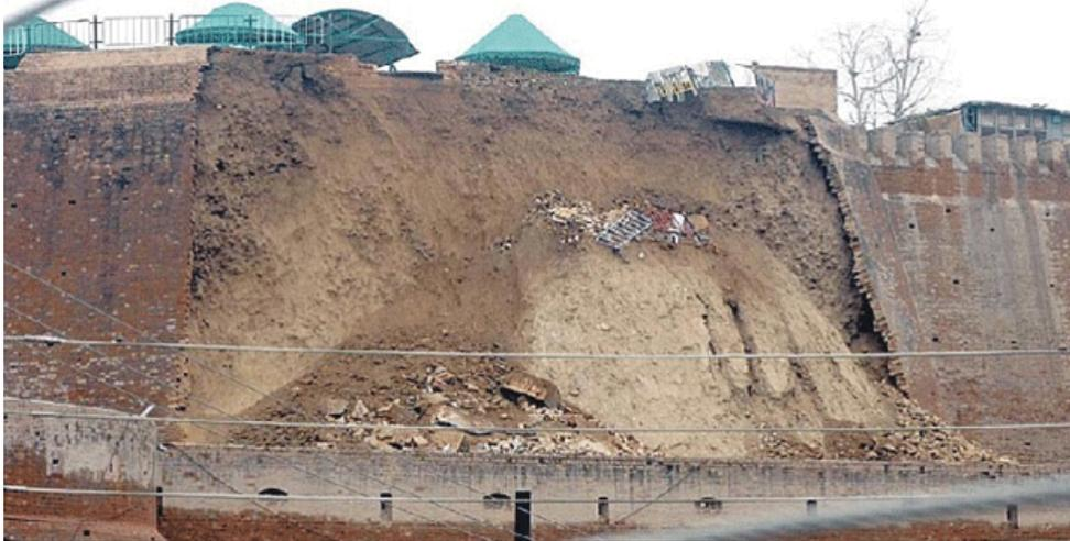
(c) Peshawar City, Fort: Collapse of masonry retaining wall and backfill sliding of Fort "Qilla Bala Hisar".
