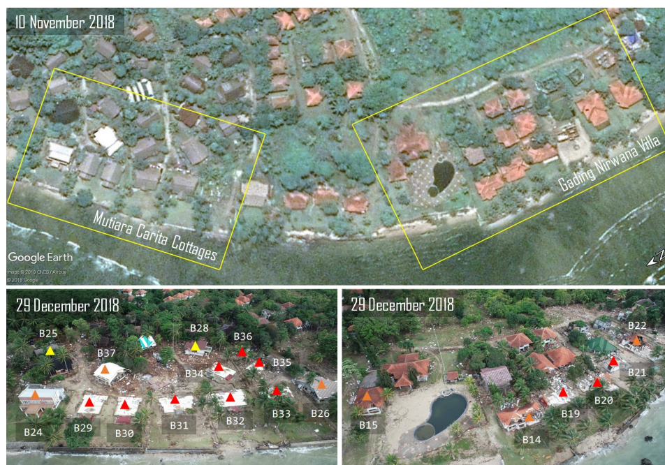
Figure 6. Aerial view of land destruction in Mutiara Carita Cottages and Gading Nirwana Villa, Banten.
