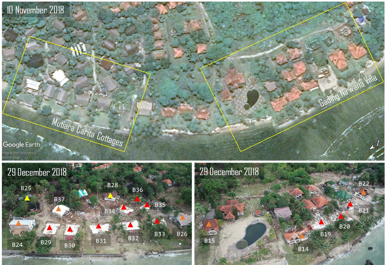
Figure 6. Aerial view of land destruction in Mutiara Carita Cottages and Gading Nirwana Villa, Banten. The upper figure was adopted from Google Earth.
