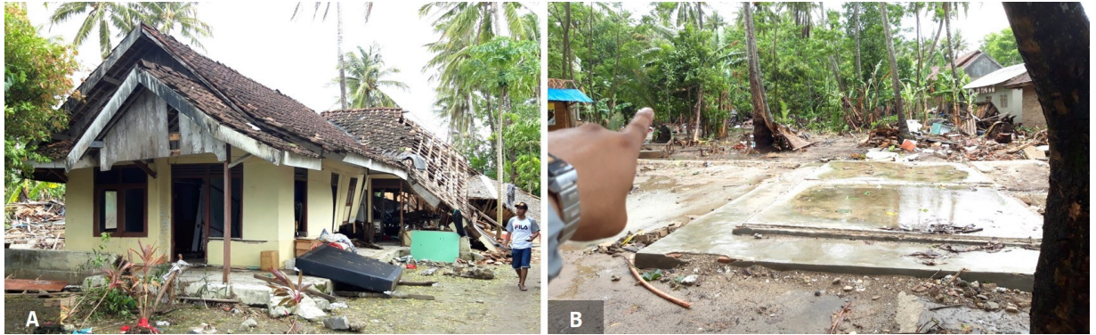
Fig. 13. Examples of damages at wooden houses: (a) major damages and (b) complete damage/washed away.
