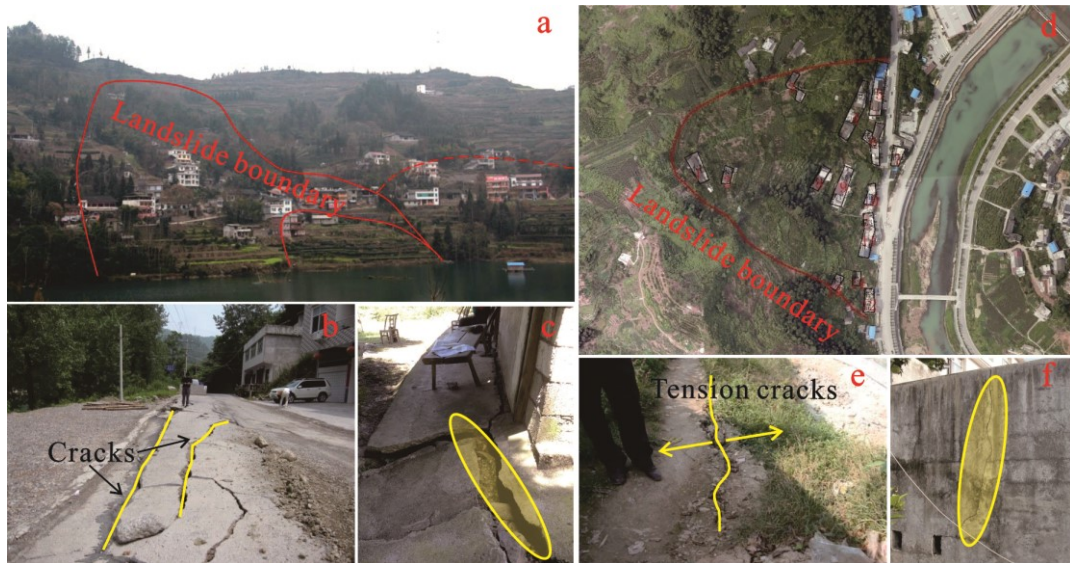
Fig. 7 The deformation of the landslides in the study area: (a) The topography of landslide (see Fig. 6 (a) for location). (b)The cracks on the road. (c) The uplift of the ground. (d) The topography of landslide (see Fig. 6 (a) for location). (e) The tension cranks on the ground. (f) The cracks on the building.
