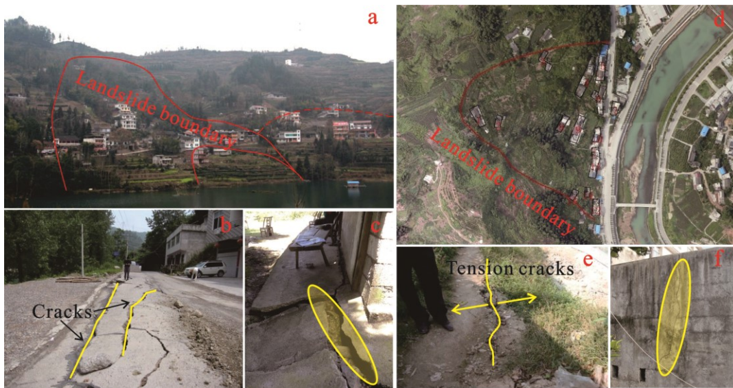
Fig. 7 The deformation of the landslides in the study area: (a) The topography of SLHL (see Fig. 6 (a) for location). (b)The cracks on the road of SLHL. (c) The uplift of the ground of SLHL. (d) The topography of HEHL (see Fig. 6 (a) for location). (e) The tension cranks of the ground on HEHL. (f) The cracks of the building of HEHL.
