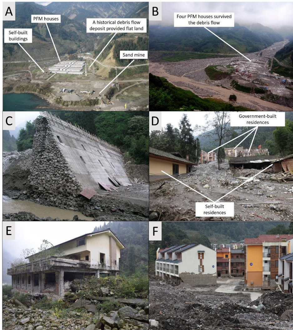
Figure 8: Losses caused by the Aug 14, 2010 debris flows. The locations of the examples are shown in Figure 8. A: The temporary settlement at the Bayi sub-catchment outlet in 2009 (Luo et al., 2010); B: The shelters destroyed by a debris flow from the Bayi sub-catchment (Luo et al., 2010); C: One of the two under designed check dams in Bayi sub-catchment which were destroyed (Liu, 2010); D: Residences reconstructed on old debris flow deposits were damaged; E: A hotel beside the Longxi River was struck; F: government-built apartment buildings beside the river were damaged.
