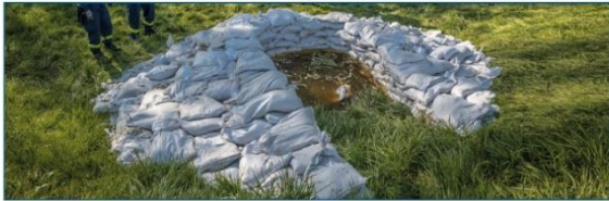
Figure 3: Dyke defence measures for a saturated dyke over an extensive are (load drain) and for heavy punctual exit of seepage (temporary ring dam). Sandbagging (left) and corresponding SBRs (right).
