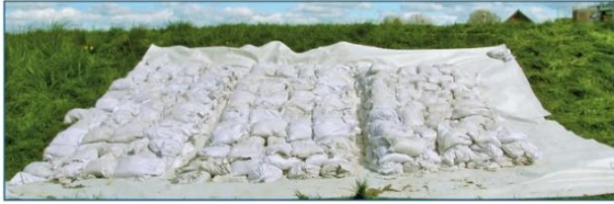
Sandbag load drain
