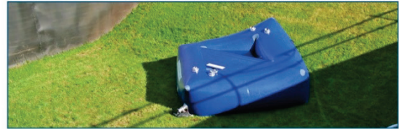
Figure 3: Dyke defence measures for a saturated dyke over an extensive are (load drain) and for heavy punctual exit of seepage (temporary ring dam). Sandbagging (left) and corresponding SBRs (right).
