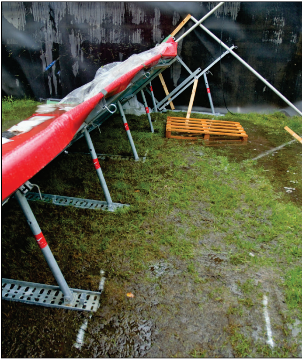
Figure 9: Supporting columns sunk into the saturated foundation soil while damming (aqua defence).
