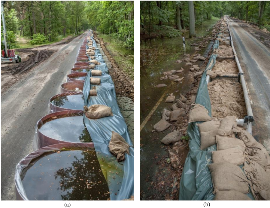
Figure 4: SBRs near Gartow (Lower Saxony, Germany) after the Elbe flood in 2013. (a) AQUARIWA, (b) Quick Damm type E.
