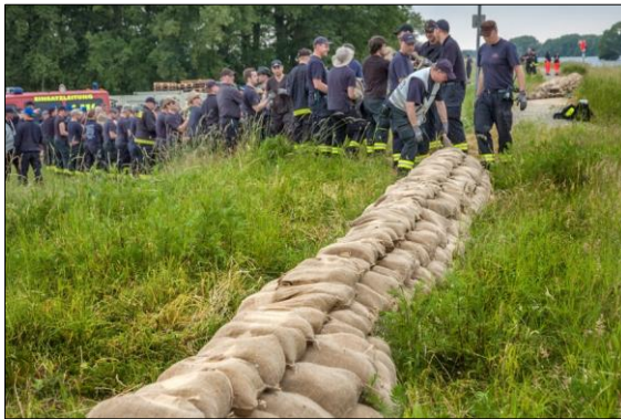
Figure 2: Firemen during the Elbe flood in 2013. Setting up a sandbag dam to raise a dyke.
