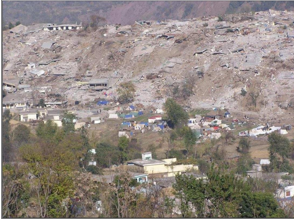
Figure 1: Impact of topography on building damages during 2005 Kashmir earthquake in Balakot (Pakistan). It can be observed that the building on ridge are completely destroyed while those at the ridge toe are still intact, despite the fact that building material and construction was similar.
