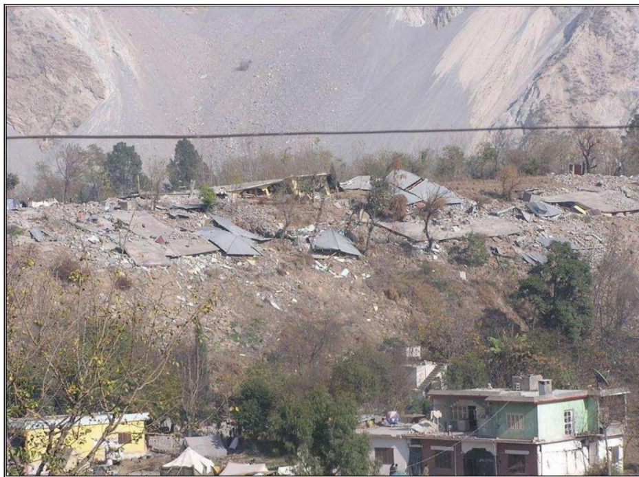
Figure 2: Impact of topography on building damages during 2005 Kashmir earthquake in Muzaffarabad (Pakistan). Same observation as in Figure 1.
