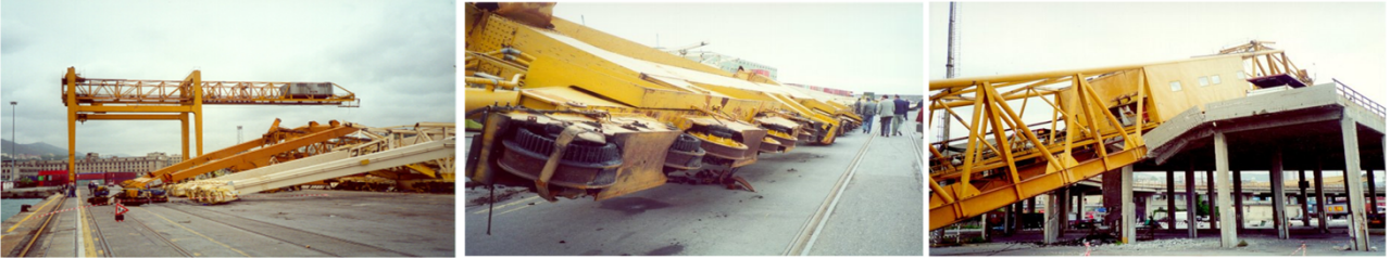
Figure 3: Damages caused by the thunderstorm downburst that occurred in the Port of Genoa (Italy) on 31 August 1994 (Photos by the Authors).
