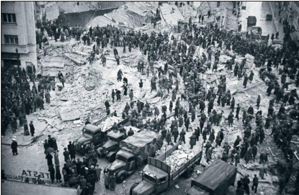
Figure 2a. The collapse of the Carlton block in Bucharest in 1940.
