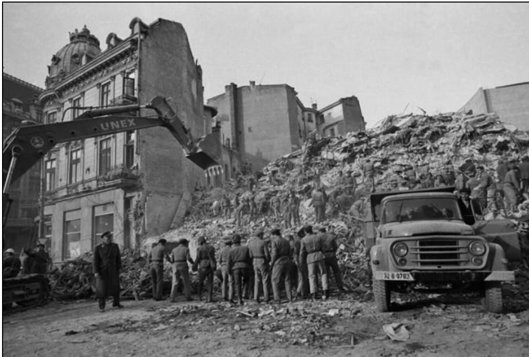
Figure 2b. The collapse of the Continental block in Bucharest's historical centre in 1977 blocked the access streets, so clearance was delayed by more than 12 hours.
