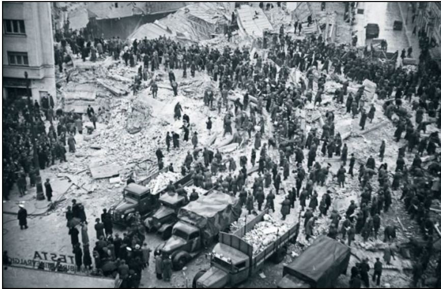
Figure 2a. The collapse of the Carlton block in Bucharest in 1940.
