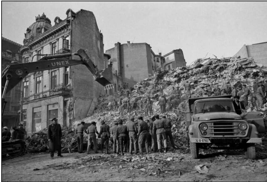
130 Figure 2b. The collapse of the Continental block in Bucharest's historical centre in 1977 blocked the access streets, so clearance was delayed by more than 12 hours; the photograph shows efforts to identify victims and property.
