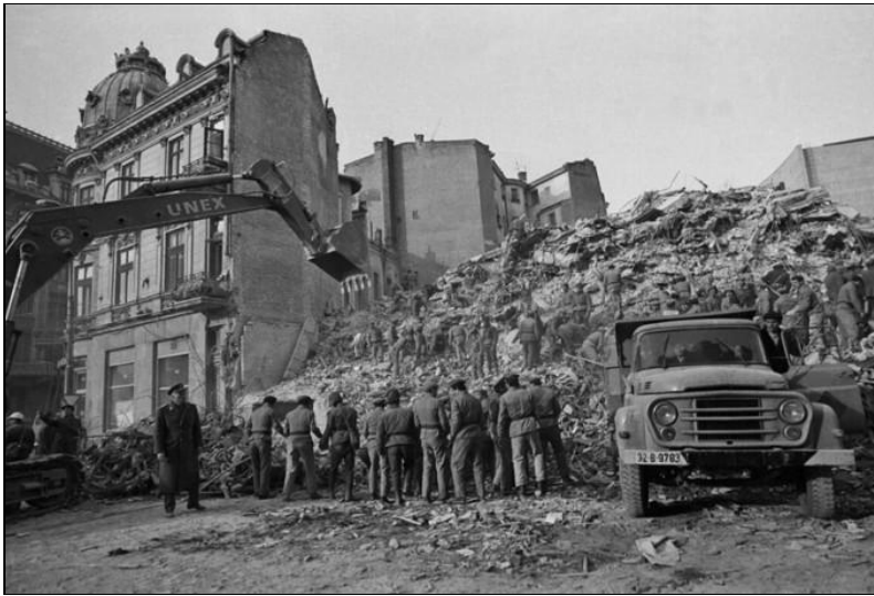
Figure 2b. The collapse of the Continental block in Bucharest's historical centre in 1977 blocked the access streets, so clearance was delayed by more than 12 hours.
