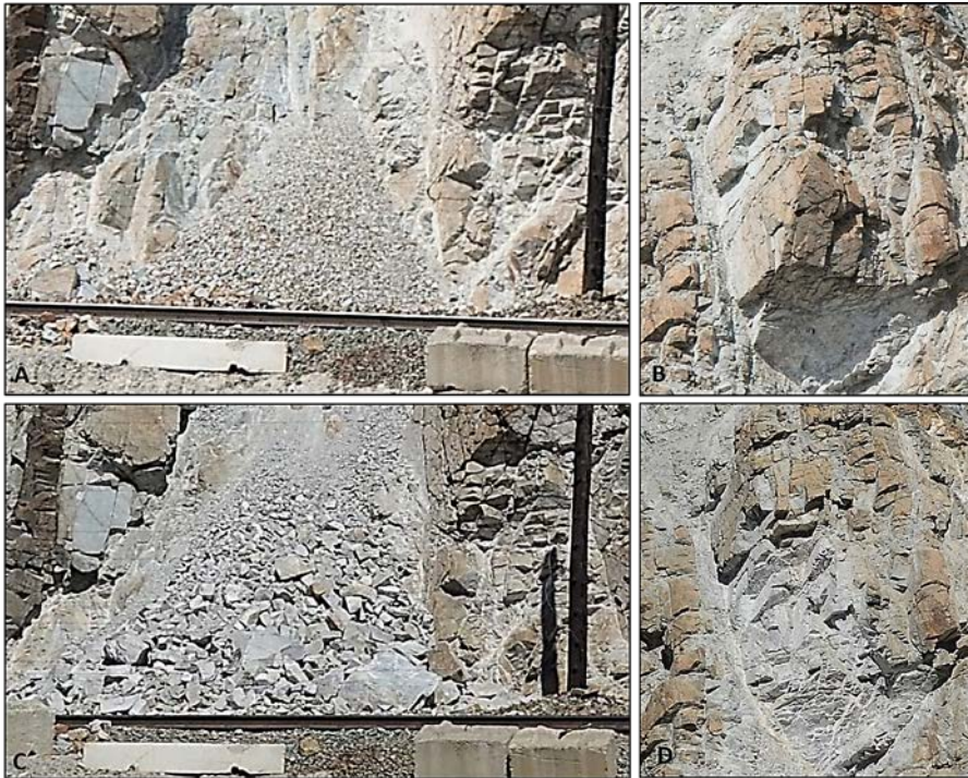
Figure 8: Before and after photos of the 24 m 3 wedge sliding event from White Canyon East, Site B. The top row of photos shows the pre-fall debris present in the track-side ditch (A), as well as the pre-fall source zone (B). The bottom row shows the post-fall accumulation in the track-side ditch (C), as well as the post-fall source zone (D). From these images we can see the heavily jointed state of the rockfall mass pre-fall and the rockfall back-scarp, post-fall. A notable increase in the quantity and size of debris fragments in the track-side ditch is visible post-fall.
