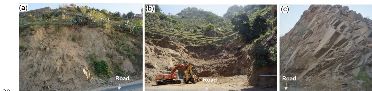
Figure 6. Landslides proximal to, and possibly triggered by, road construction. (a) Debris flow caused by failure on steep slopes intersected by roads. (b) Debris flow caused by failure of terraces constructed on steep slopes. (c) Landslide flow caused by failure on fracture planes dipping towards the road.
