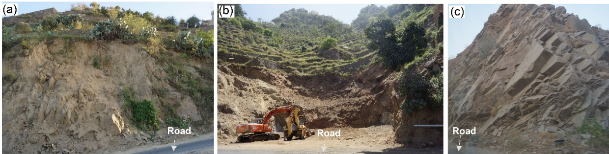
Figure 5. Landslides proximal to, possibly triggered by, road construction and intensified by rainfall (a) Debris flow caused by failure on steep slopes intersected by roads. (b) Debris flow caused by failure of terraces constructed on steep slopes. (c) Landslide caused by failure on fracture planes dipping towards the road.
