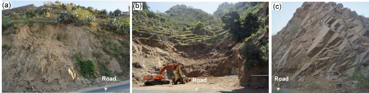
Figure 5. Landslides proximal to, possibly triggered by, road construction and intensified by rainfall (a) Debris flow caused by failure on steep slopes intersected by roads. (b) Debris flow caused by failure of terraces constructed on steep slopes. (c) Landslide caused by failure on fracture planes dipping towards the road.
