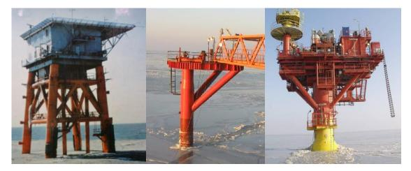
(a) Four-legged oil production platform (built in 1987); (b) One-legged auxiliary platform (built in 1999); (c) One-legged oil production platform (built in 2003).
