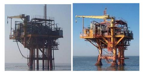
5 (d) Three-legged upright pile production platform (built in 1997); (e) Three-legged upright pile production platform with cones (built in 2000)
