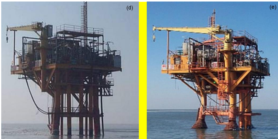
(d) Three-legged upright pile production platform (built in 1997); (e) Three-legged upright pile production platform with cones (built in 2000)
