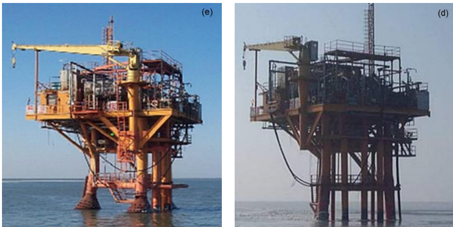
(d) Three-legged upright pile production platform (built in 1997); (e) Three-legged upright pile production platform with cones (built in 2000)
