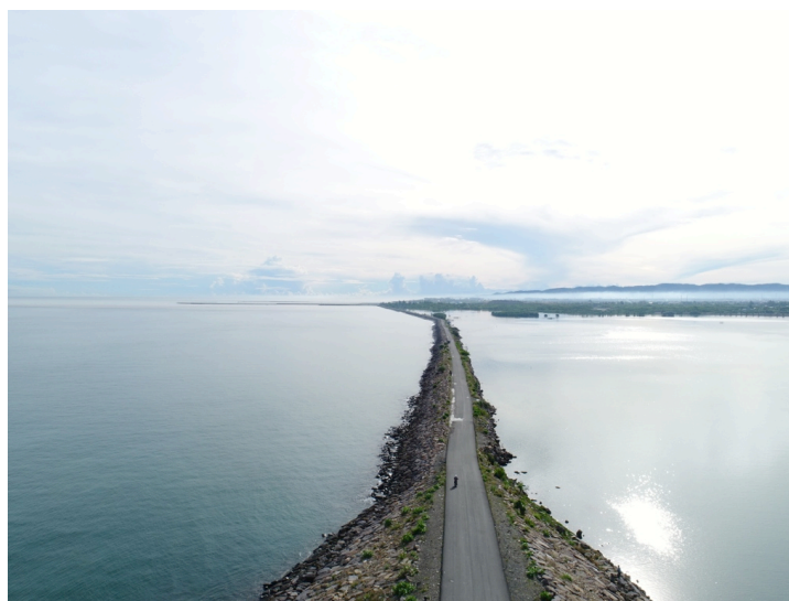
Figure 3. A 7-km embankment along the coast of Banda Aceh where a road was constructed at the leeward side of the embankment (Photo taken date, February 2018?).
