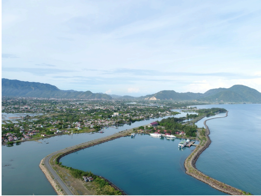
Figure 2: The situation of the coastal area of Banda Aceh based on aerial image taken in February 2018.
