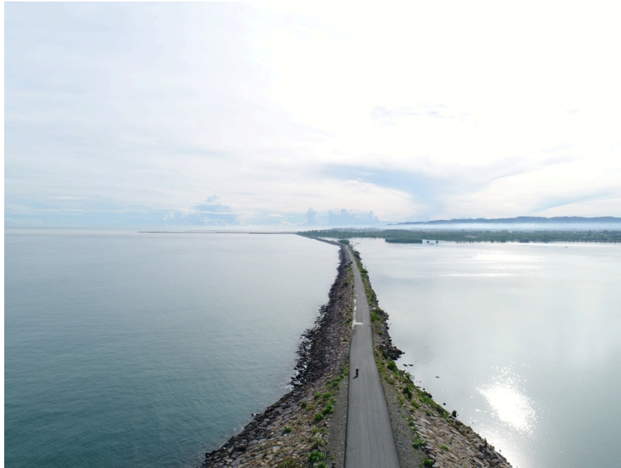
Figure 3. A 7-km embankment along the coast of Banda Aceh where a road was constructed at the leeward side of the embankment (Photo taken date: February, 2018).
