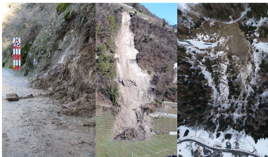
1011 Figure 8: Examples of events affecting roads. Left: small event already removed but still unstable on the unique 1012 access road to the small village of Morcles (canton of Vaud). Middle: middle event on a minor road in Ollon (canton 1013 of Vaud). Right: large event with a volume estimated at 3500 m 3 that cut on a 50 m length the international road 1014 between France and canton of Valais near the Forclaz pass (Trient). Road closure is estimated of six weeks. Images 1015 taken on 24 January 2018 after a winter storm.
