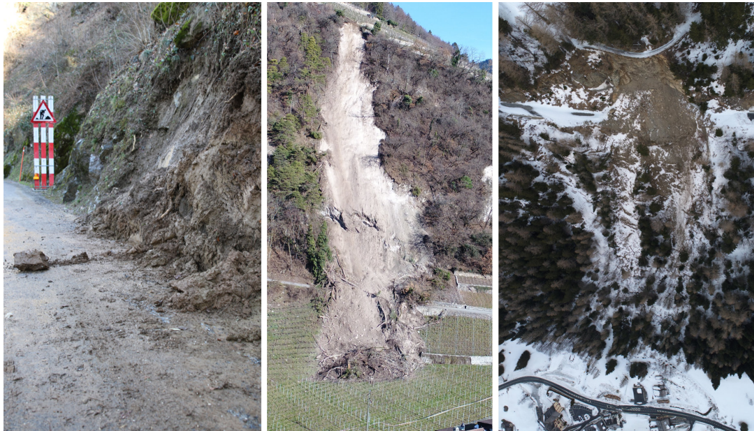
Figure 4: Examples of events affecting roads. Left: small event on the only road to the small village of Morcles (Canton of Vaud). Middle: middle-sized event on a minor road in Ollon (Canton of Vaud). Right: large event with an estimated volume of 3500 m 3 that cut a 50 m length on the international road between France and Canton of Valais near the Forclaz pass (Trient). The road closure was estimated at six weeks. Images taken on 24 January 2018 after a winter storm.
