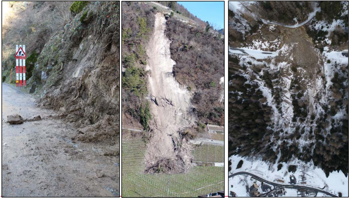
Figure 8: Examples of events affecting roads. Left: small railway classes according event already removed but still unstable on the unique access road to the small village of Moreles (canton of Vaud). Middle: middle event on a minor road in Ollon (canton of Vaud). Right: large event with a volume estimated at 3500 m 3 that cut on a 50 m length the international road between France and canton of Valais near the Forclaz pass (Trient). Road closure estimated of six weeks. Images taken on 24 January 2018 after a winter storm processes.
