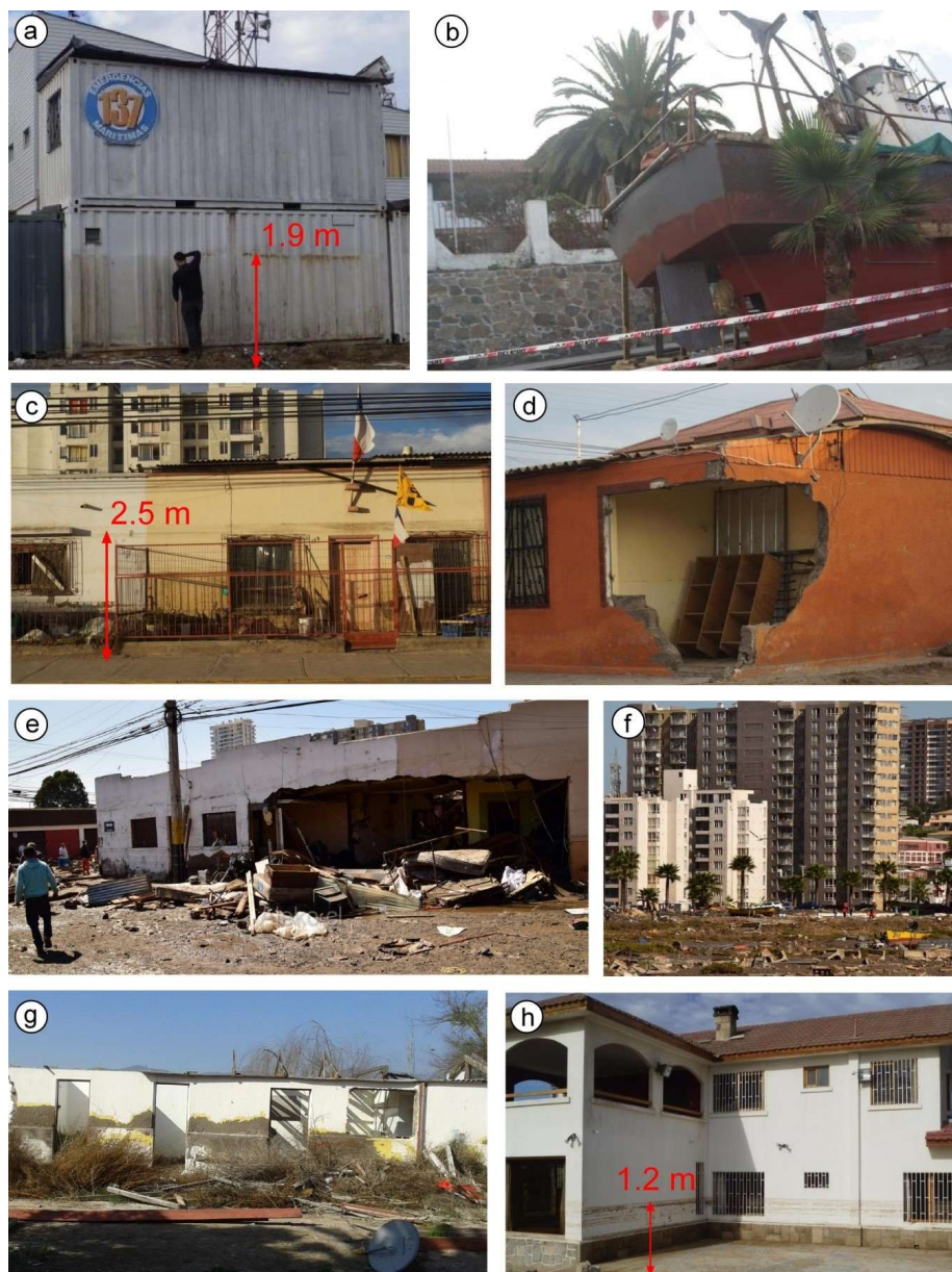
Figure 4: a) Building with average RVI score in the first coastline with flood heights of 1.9 m after the 2015 tsunami in Coquimbo Port (sector 1); b) Movable objects impacting residential buildings after the 2015 tsunami; c) High vulnerability building with more than 50% of its infrastructure flooded; d) High vulnerability building with its damaged infrastructure after the 2015 tsunami; e) Very high vulnerability building that resulted in non-repairable damage after the 2015 tsunami; f) Modern buildings with minor vulnerability RVI score; g) Very high vulnerability building highly affected by the tsunami in La Cantera sector; h) Not open plan ground floor.
