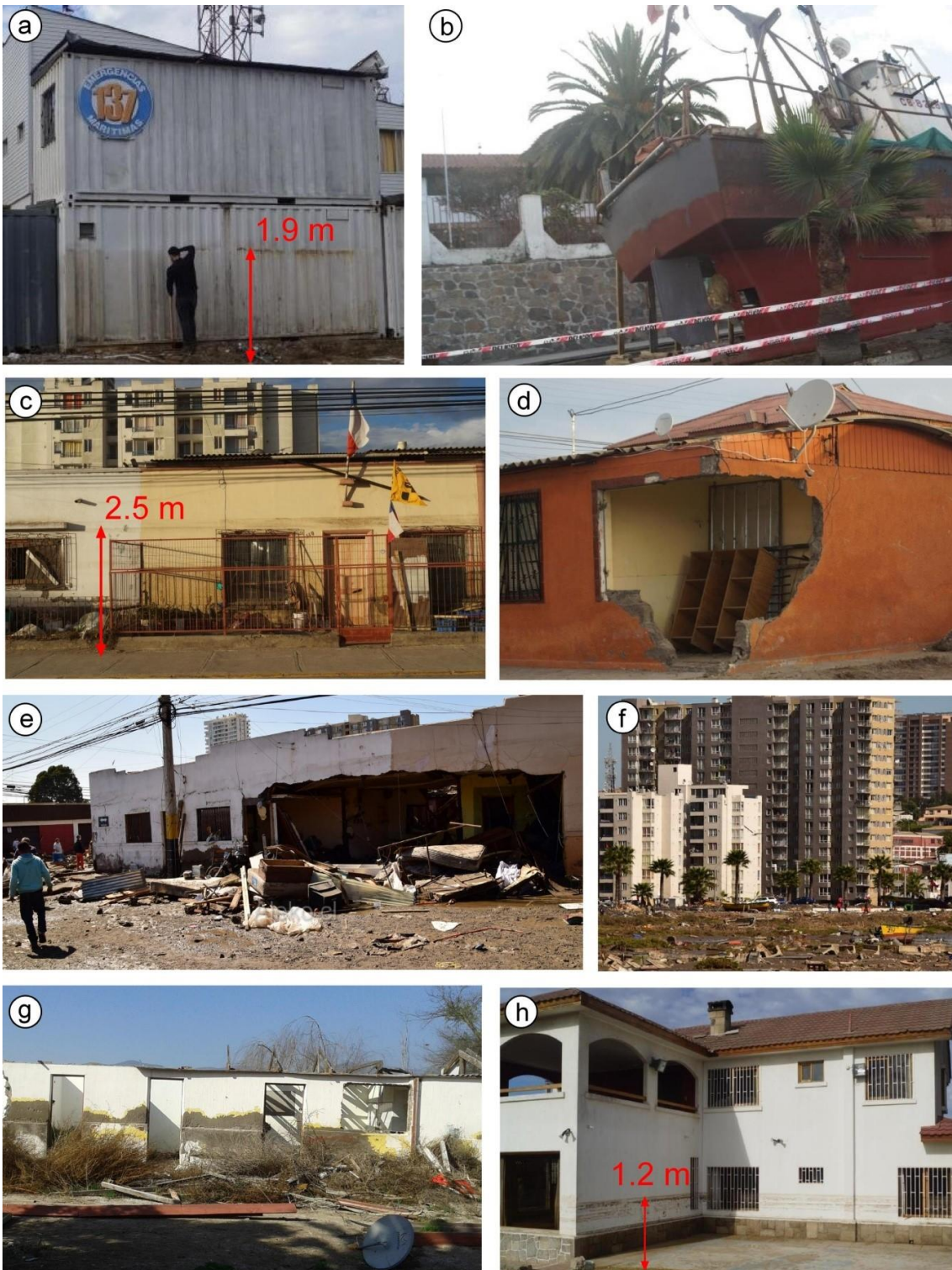
5 Figure 4: a) Building with average RVI score in the first coastline with flow depths of 1.9 m after the 2015 tsunami in Coquimbo Port (sector 1); b) Movable objects impacting residential buildings after the 2015 tsunami; c) High vulnerability building with more than 50% of its infrastructure flooded; d) High vulnerability building with its damaged infrastructure after the 2015 tsunami; e) Very high vulnerability building that resulted in non-repairable damage after the 2015 tsunami; f) Modern buildings with minor vulnerability RVI score; g) Very high vulnerability building highly affected by the tsunami in La Cantera sector; h) Not open plan ground floor.
