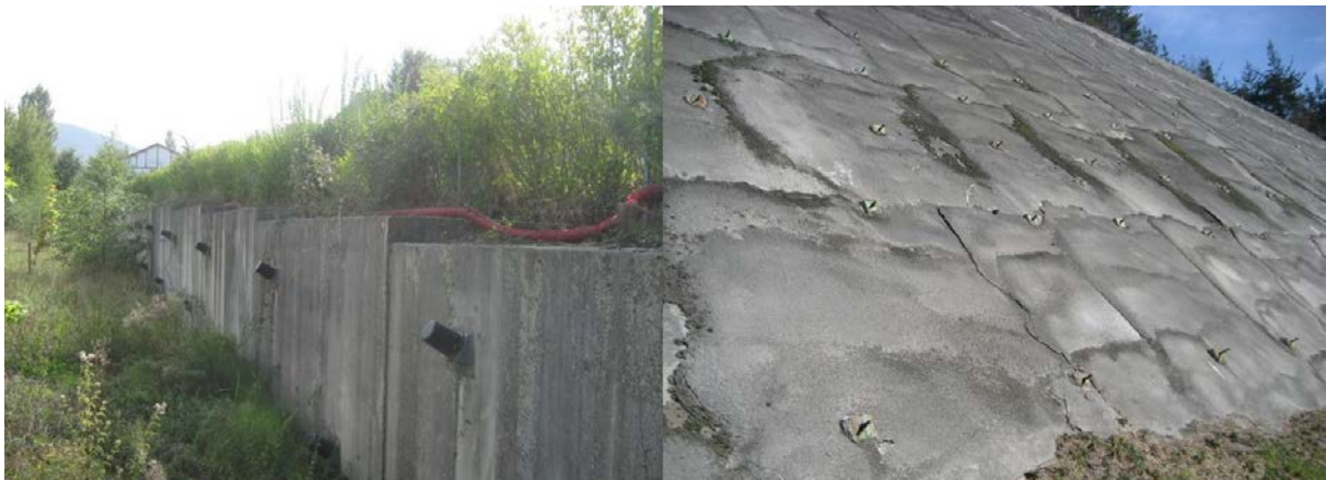
Figure 8: (left) PoR P2A of the road AP-8-1-1 (from km 77.140 to 77.210) where the crest of the slope and the retaining wall with anchors is seen; (right) C8A of the road G-2634 (32.980 to 33.150) with gunite, rock bolts, and anchors.
