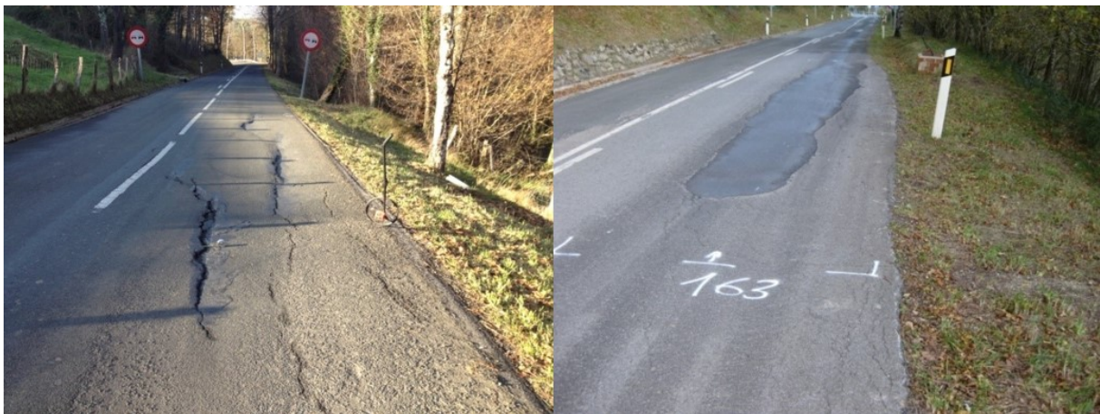
Figure 9: Road sections situated within slow moving landslides, with damage: (left) PoR C3C of the road GI-2133 (from km 8.280) with observed deformations and cracks on the road pavement; (right) PoR C9G of the road GI2637 (from km 17.891 to 18.220) showing minor cracks already sealed.
