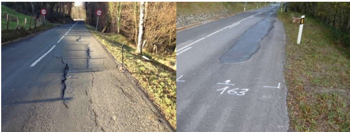
25 Figure 9: Road sections situated within slow moving landslides, with damage: (left) PoR C3C of the road GI-2133 (from km 8.280) with observed deformations and cracks on the road pavement; (right) PoR C9G of the road GI2637 (from km 17.891 to 18.220) showing minor cracks already sealed.
