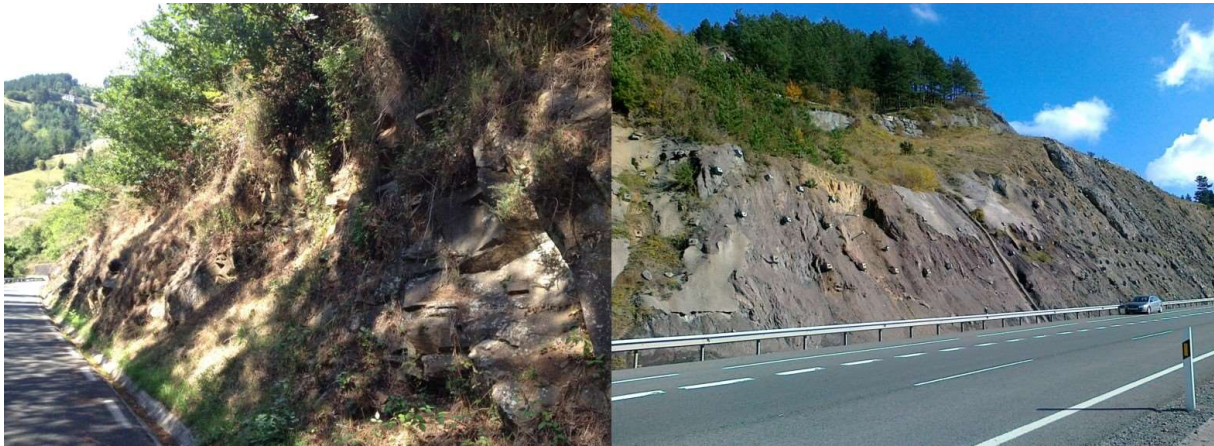
5 Figure 7: (left) PoR L1C of the road GI-3324 (from km 0.700 to 1.450), without protection measures; (right) PoR P4C of the road N-1 (km 407.395 to 407.680) with protection measures.
