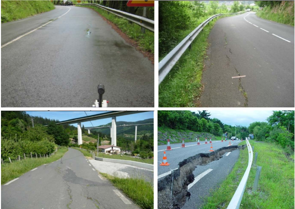
Figure 5: The four damage levels identified at the roads of Gipuzkoa: (top-left) No/Slight damage, (top-right) Moderate damage, (down-left) Severe damage, and (down-right) Partial/total destruction.
