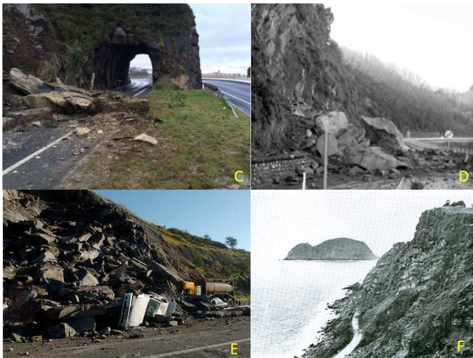
Figure 3: Examples of rockfall magnitudes (C, D, E, and F) in the study area, in relation to the classes of Table 2 (source: photo D, E: Javi Colmenero; F: Servicio Geológico de Obras Públicas)
