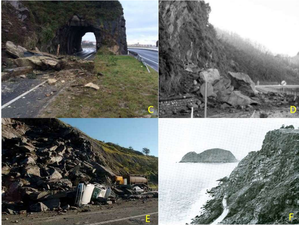
Figure 3: Examples of rockfall magnitudes (C, D, E, and F) in the study area, in relation to the classes of Table 32 (source: photo D, E: Javi Colmenero; F: Servicio Geológico de Obras Públicas)
