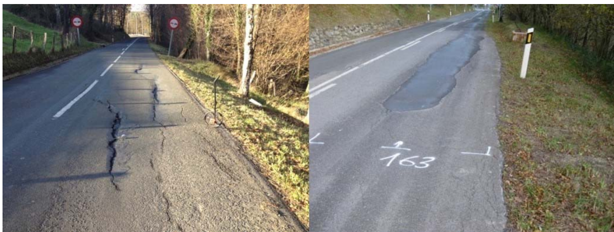
Figure 9: Road sections situated within slow moving landslides, with damage: (left) PoR C3C of the road GI-2133 (from km 8.280) with observed deformations and cracks on the road pavement; (right) PoR C9G of the road GI2637 (from km 17.891 to 18.220) showing minor cracks already sealed.
