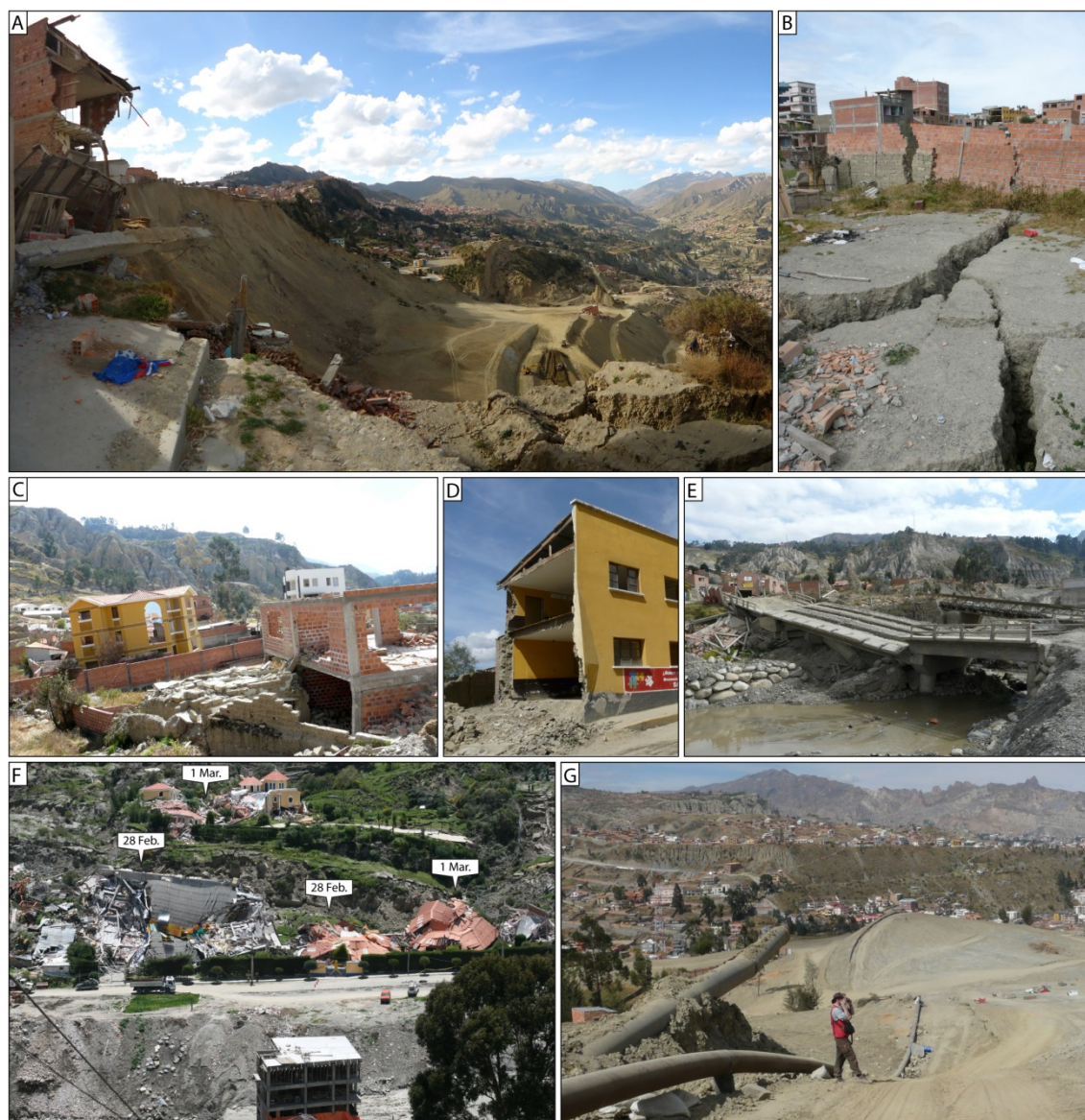
Figure 5. Impacts of the 2011 Pampahasi landslide. A. Headscarp (80 m height) along the east margin of Pampahasi Plateau (note excavator and trucks in lower middle ground for scale). B. Ground fissures in the northern part of the lower landslide mass. The wall in the background is ~2 m high. C. Back-tilted houses and apartment buildings on the northern part of the lower landslide mass (movement was from left to right). D. Community building with collapsed wall on the northern part of the lower landslide mass. E. Bridge across Río Irpavi that was deformed and shifted from its footings on 28 February near the centre of the landslide toe. F. Buildings on the southern part of the toe of the landslide (that collapsed on 28 February and 1 March (dates of collapse shown; photo by M.A. Guzmán, 2 March 2011)). G. Water service line ruptured by the landslide (upper pipe) and replacement water service line (lower pipe). See Figures 2B and 7C, D for locations of photographs. Photos taken by N.J. Roberts in May 2011 unless otherwise indicated.
