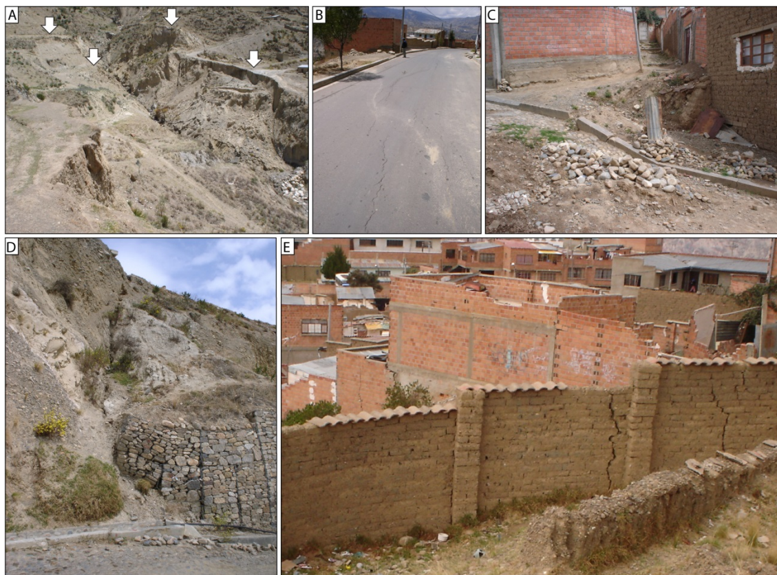
Figure 4. Field evidence of pre-failure creep in what would become the head region of the 2011 Pampahasi landslide. A. Small recent slumps (arrows) along Río Chujilluncani, ~400 m downslope from the east margin of Pampahasi Plateau. B. Minor cracking and centimeter-scale vertical offset of a paved road about 200 m east of, and 75 m below, the east margin of the plateau. C. Unpaved road with ~1 m displacement near the 2011 headscarp. D. Vertical offset along a gully ~75 m from the future south lateral margin of the 2011 landslide. The side of the gully nearer the middle of the 2011 landslide (right of the photo) has dropped ~0.5 m relative to the adjacent slope, causing deformation of the gabions and curb in the foreground. E. Cracks in an adobe wall (right foreground) and brick house (left middle ground) ~50 m downslope of the east margin of the plateau, corresponding to the middle of the 2011 landslide headscarp. See Figures 2A and 7A, B for locations of photographs. Photos taken by R.L. Hermanns in October 2005.
